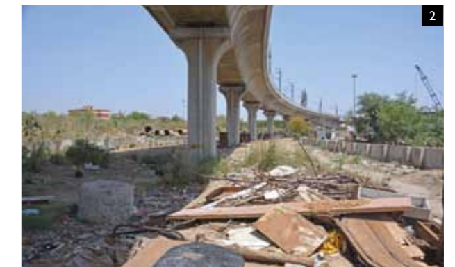
View showing space below Metro corridor
