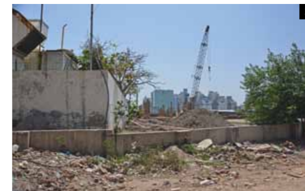
View showing area behind petrol pumps
